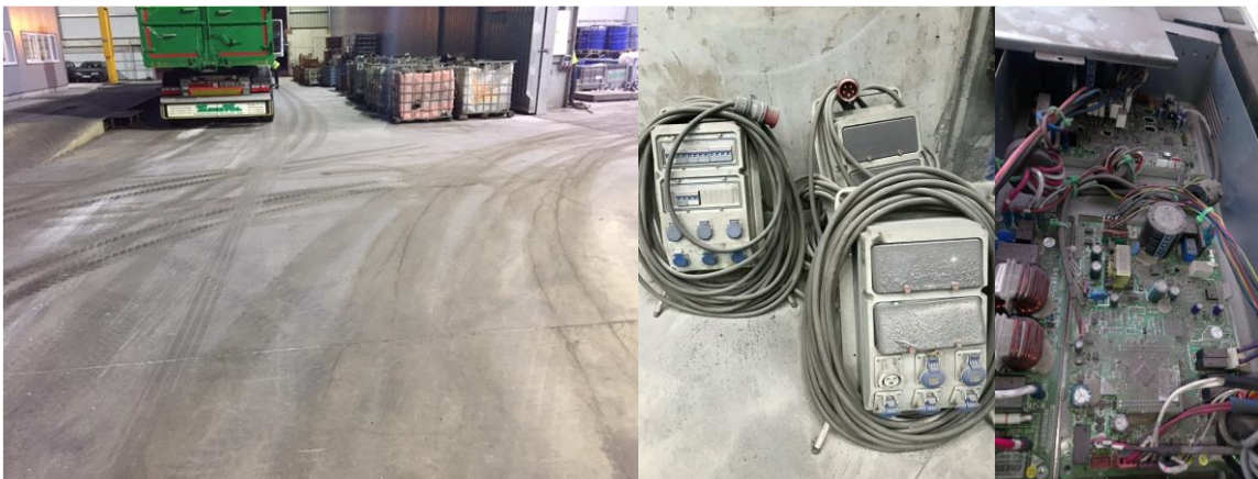
Source: Port authority of Bilbao; examples of deteriorated surfaces and equipment.
